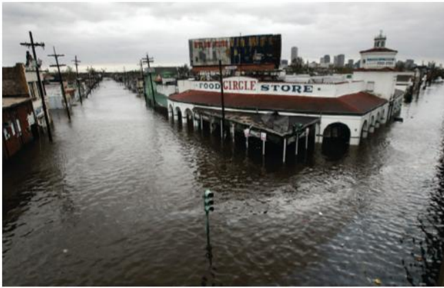
Figure 5.32 Destruction caused by Hurricane Katrina, New Orleans, 2005
