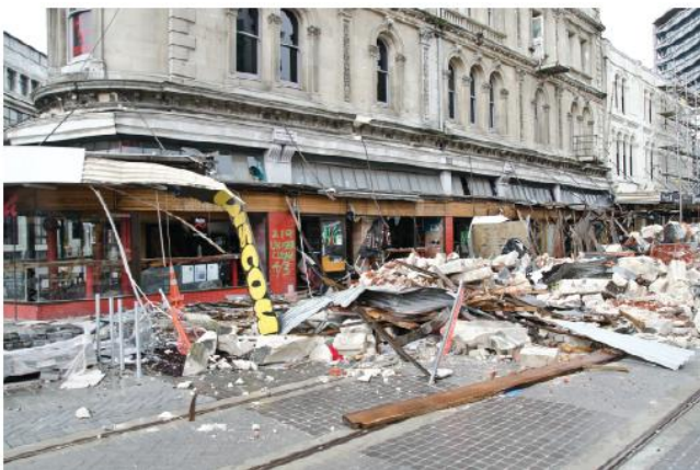
Figure 5.28 Devastation caused by the Christchurch earthquake, New Zealand, 2011
