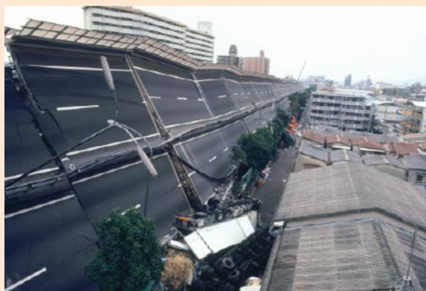
Figure 5.44 Damage caused by the Great Hanshin Earthquake, Kobe, Japan, January 1995
