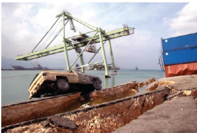
Figure 5.26 Devastation caused by the Haiti earthquake, January 2010
